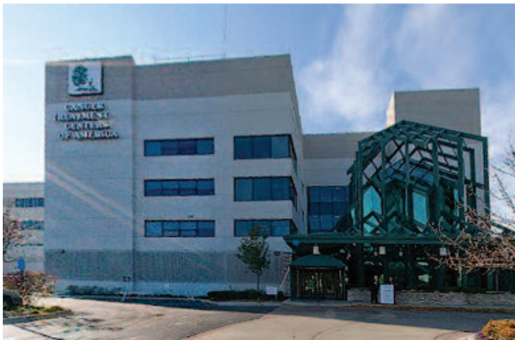
CTCA headquarters outside Chicago.
